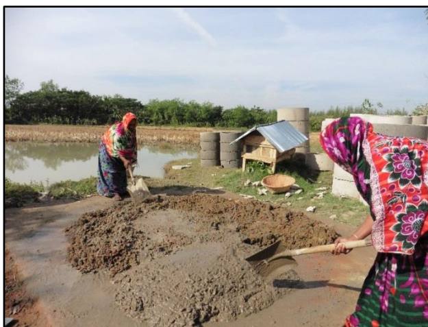
Nargis and Parul mixing concrete
